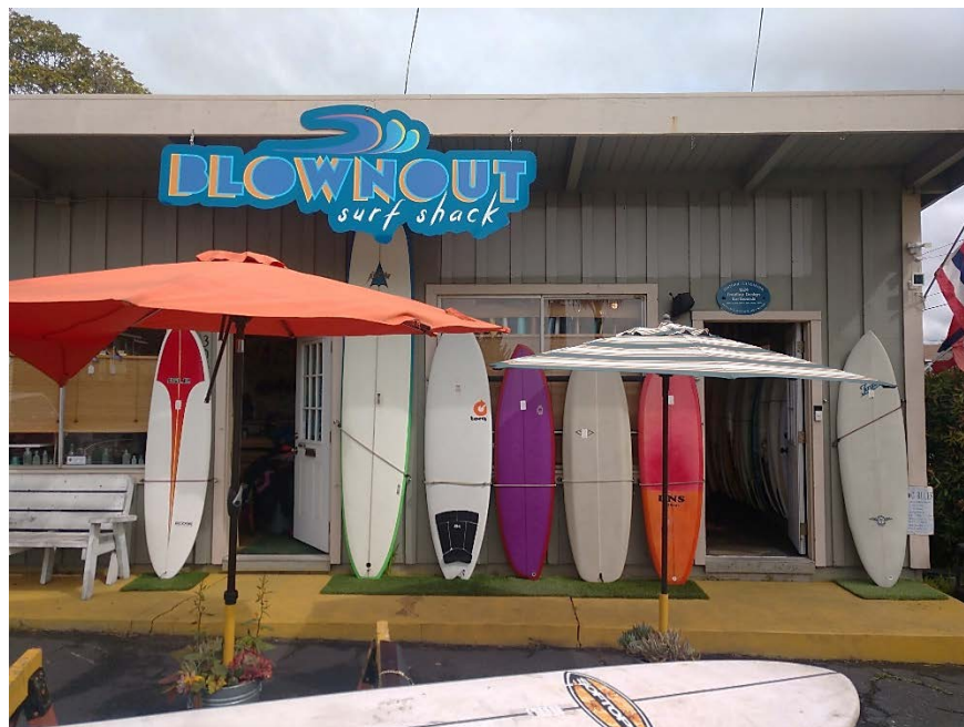
Front view of building
