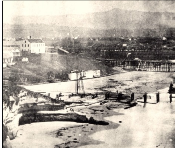
Railroad Wharf under construction, 1875. Powder Mill Wharf in distance. (Harold van Gorder collection)
