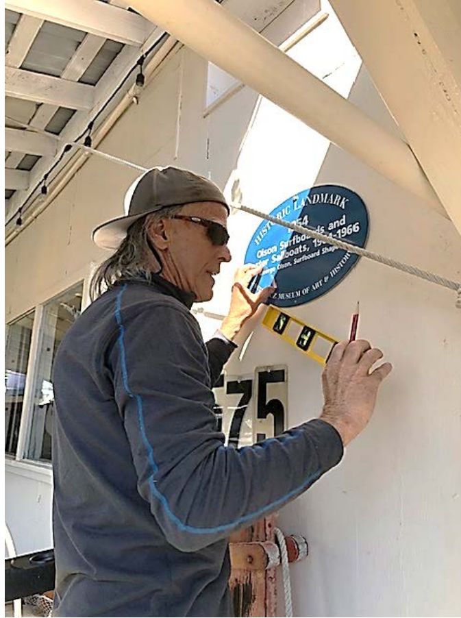
Randy leveling the Blue Plaque for installation
