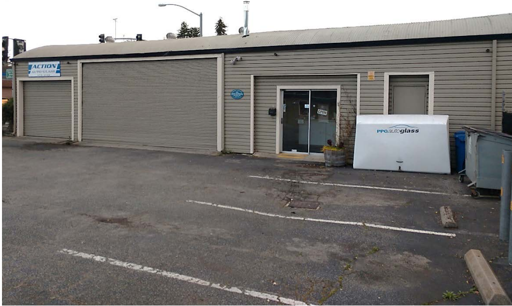
Side view of old former Yount Surf Shop
